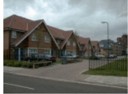
Family Housing, Old Kenton Lane
